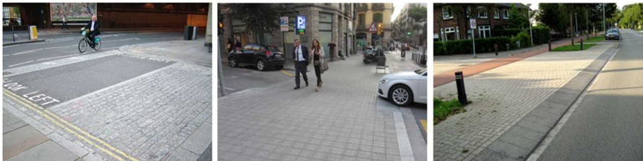
Figure 7.a Examples of raised crossings at junctions on main roads meeting minor roads, emphasising the legal priority of pedestrians and cyclists going straight ahead over entering/exiting motor traffic, and slowing same motor traffic in the process.
