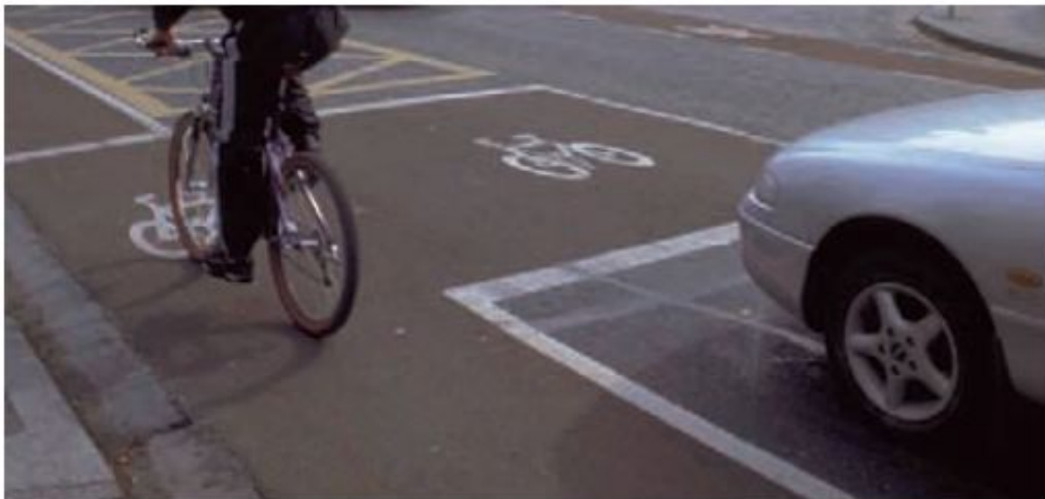
Figure 5.6 Image from NCM showing advanced stacking location/advanced stop line for cyclists.
