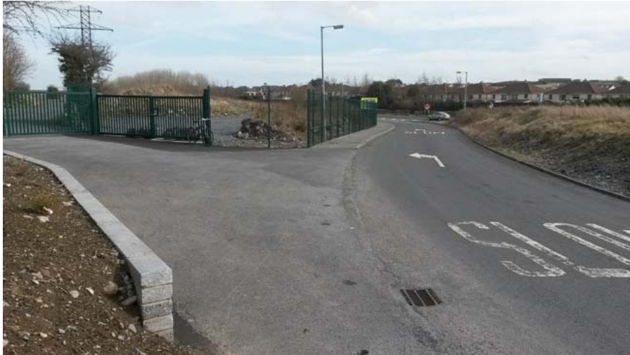
Figure: Junction of internal road within race course and Ballybane Industrial estate – showing location relative to N6 slip road.
