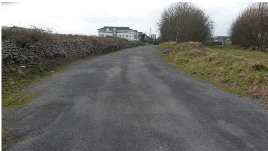
Figure: Internal road within race course looking back at Ballybane Industrial estate.
