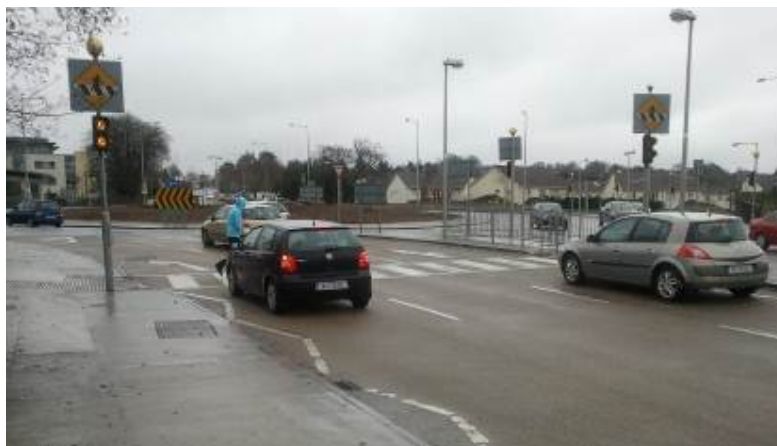
Figure: Limerick: Zebra crossings on Groody roundabout
