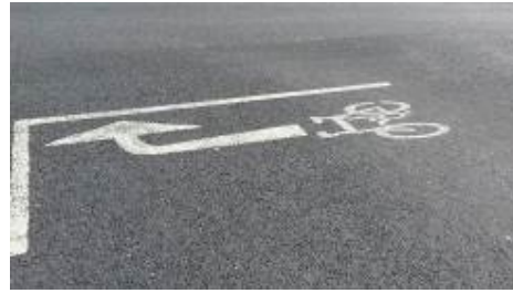
Figure: Galway, junction at NUI, Galway showing traffic signals with bike box and cycle lane before the red overlay was applied. The main lanes have sensor loops for cars but cycle lane and bike box have no sensors for cyclists. The buried wires cross the cycle track but there is only a rectangular sensor loop for motor vehicles.
