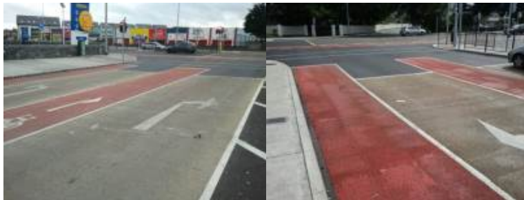
Figures: Galway junctions showing traffic signals with sensor loops for cars but not for cyclists. If only cyclists are present, the lights will stay red.
