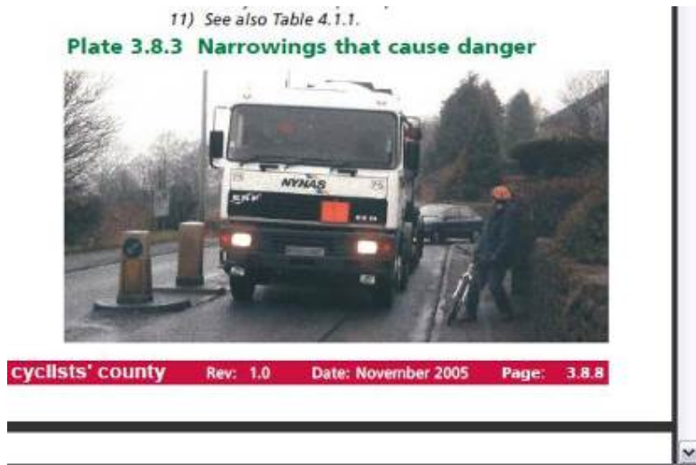
Figure: Illustration from UK design manual showing hostile pinch point. Source: Lancashire a cyclists' county.
