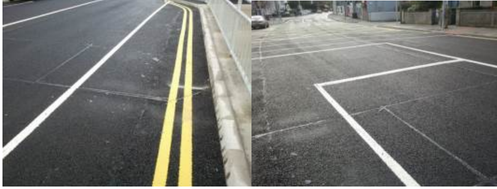
Figure: Galway, junction at NUI, Galway showing traffic signals with bike box and cycle lane before the red overlay was applied. The main lanes have sensor loops for cars but cycle lane and bike box have no sensors for cyclists. The buried wires cross the cycle track but there is only a rectangular sensor loop for motor vehicles.
